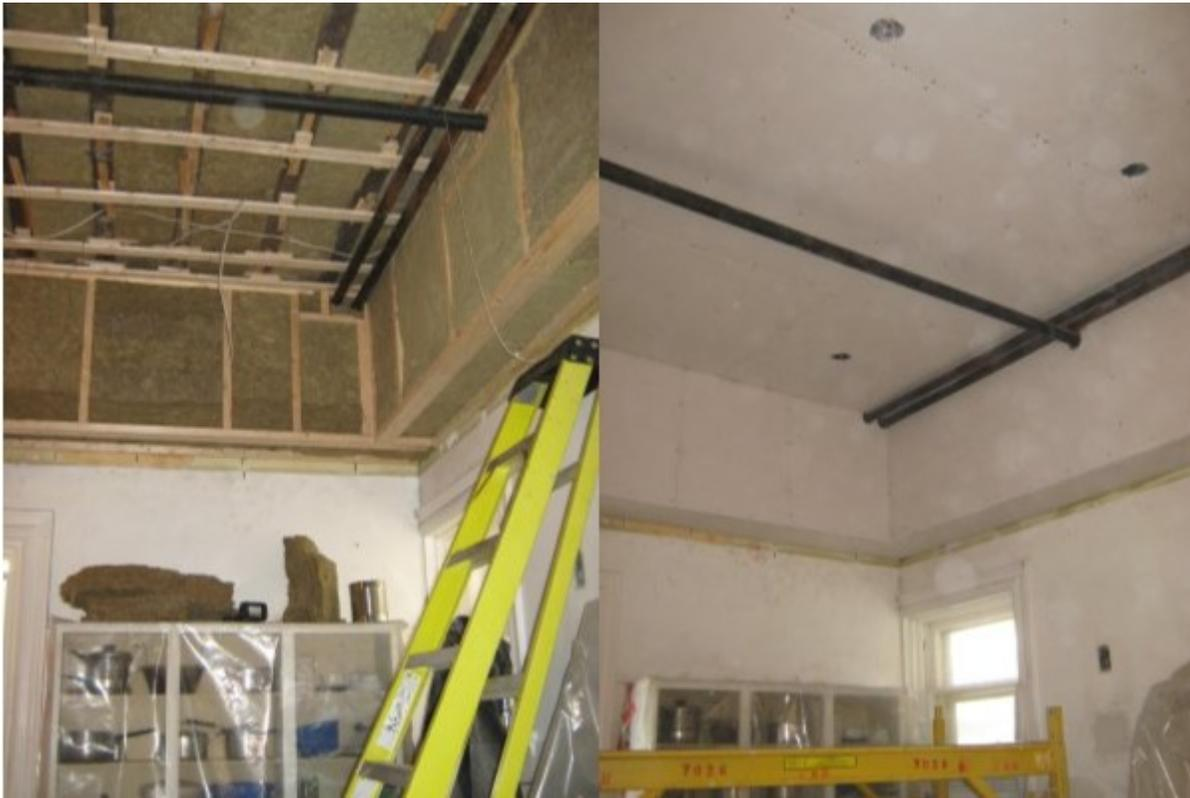
*Bulkhead built around perimeter of ceiling and drywall installed*
