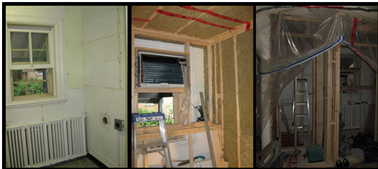
Construction photographs of the Walk-in Cooler in the Kuin (kitchen)
