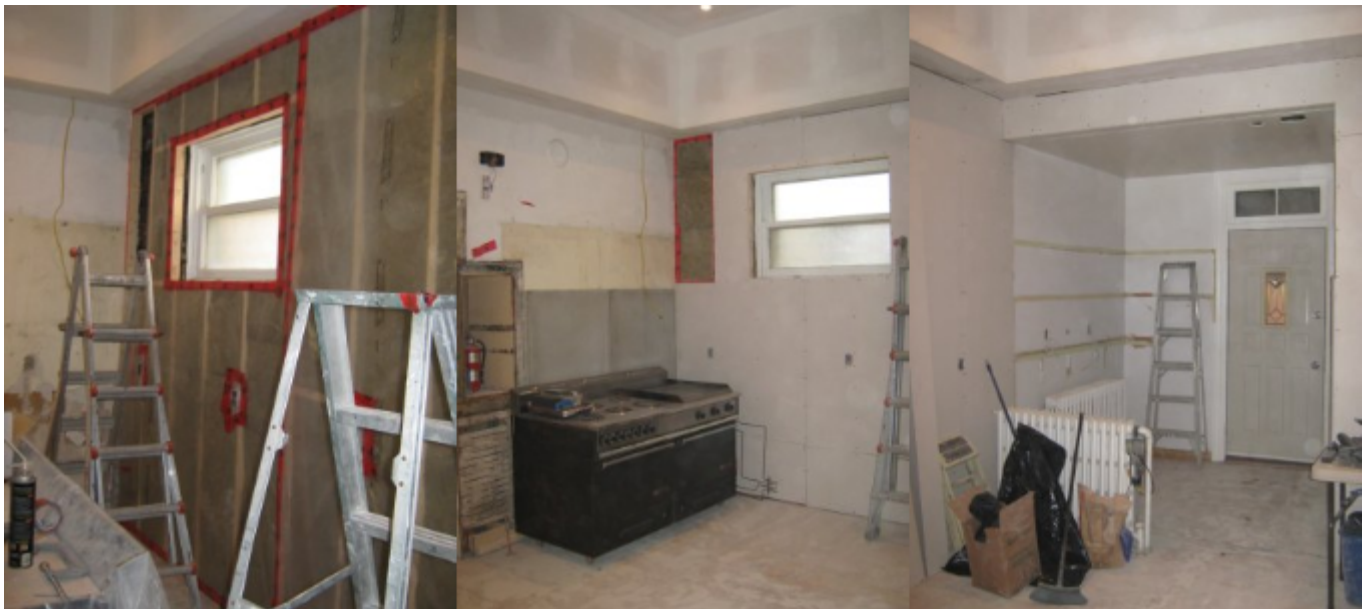
Images of Kuin walls in process
