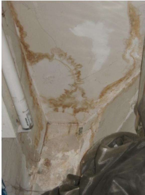
The image above shows the damage to the ceiling in Shikai sensei's room from several years of leaks in the bay window. Other roofs of the building are also in need of repair. During
